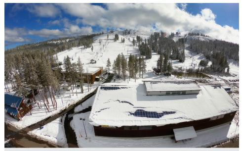
Sized appropriately, Boreal's solar system was designed to handle 356 pounds per square foot of roof snow -- far more than the average snowstorm might deliver in any given day. This design reduces risk of potential panel damage before maintenance teams can remove accumulated ice and snow, and ensures optimum production of clean solar energy.
